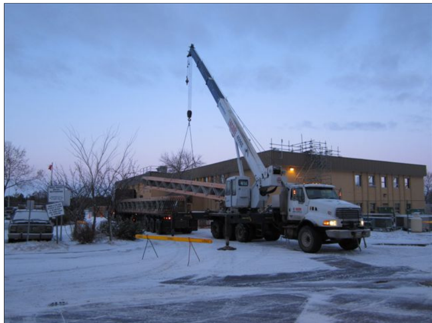
Delivery of Trusses
